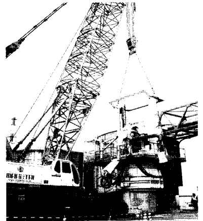
RCD施工風景
