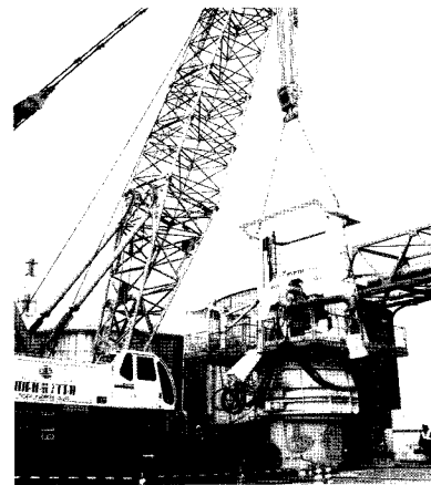
RCD施工風景
